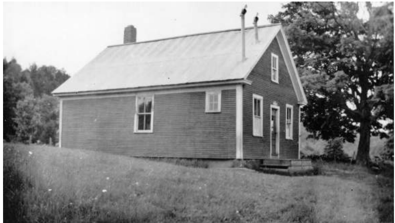
North Bridgewater School
