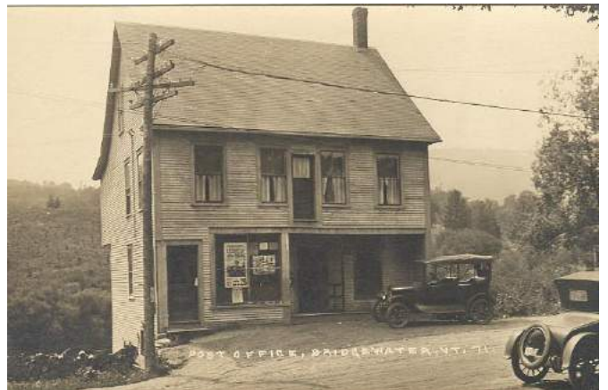
Bridgewater Village Post office 1921
