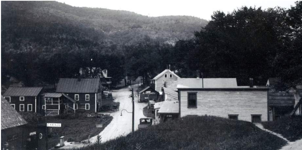
Bridgewater Corners looking west from the Upper Road showing Miner Garage on the left with Corners Store further along Route 4 on left
